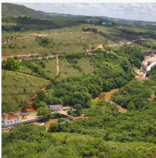
AMG hydroelectric plant in Brazil
